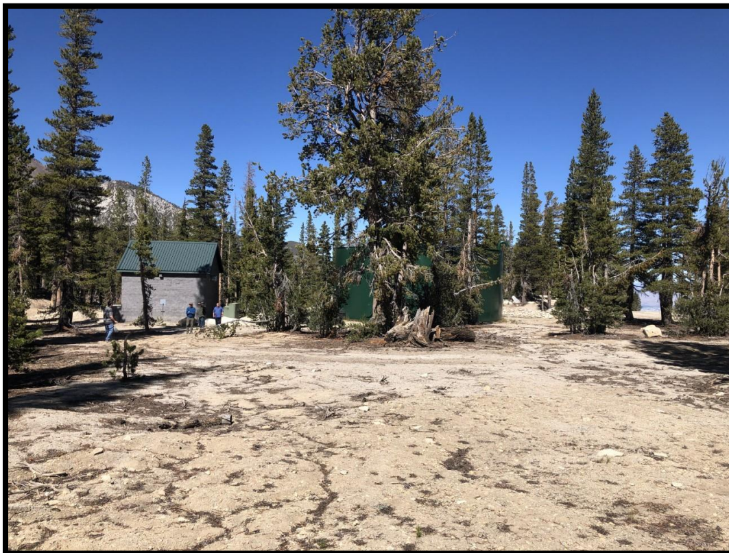
Photo looking north at the proposed tank site as well as the existing 500,000-gallon water tank and maintenance building
